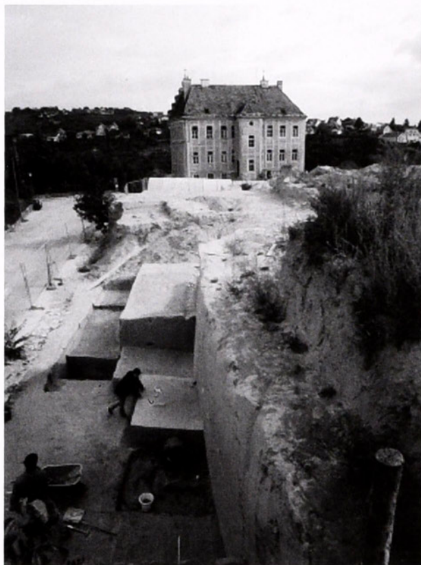
Figure 1. Krems/Hundssteig, excavation area (2001). Photo: PK, ÖAW.
